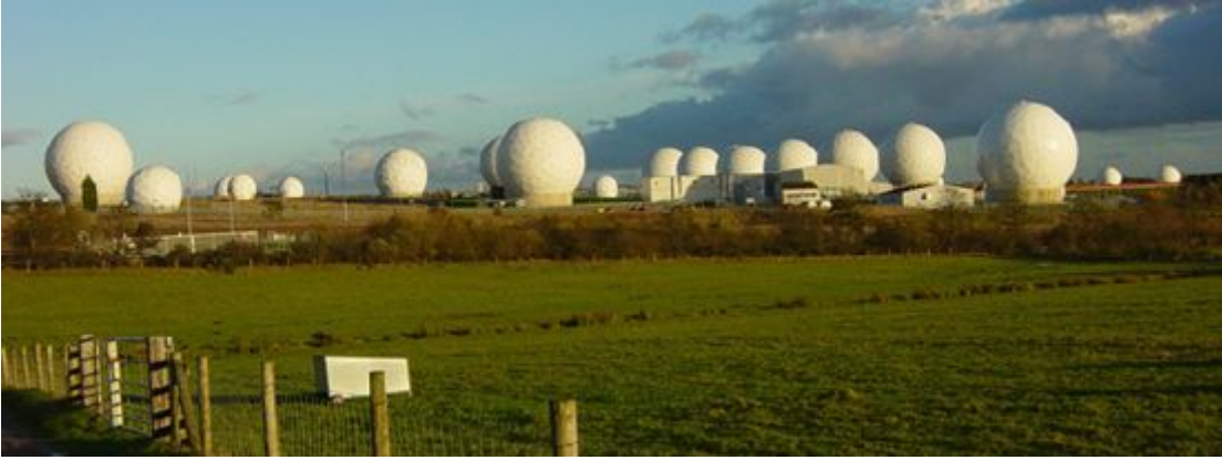
Radomes at Menwith Hill, a Royal Air Force station in North Yorkshire, England. The antenna systems operated by British and U.S. intelligence services partly function as a communications intercept for intelligence gathering and partly as a satellite ground station. The site is considered the largest electronic monitoring station in the world. Photo: Matt Crypto (cropped), November 2005. Source: Wikimedia Commons, public domain
